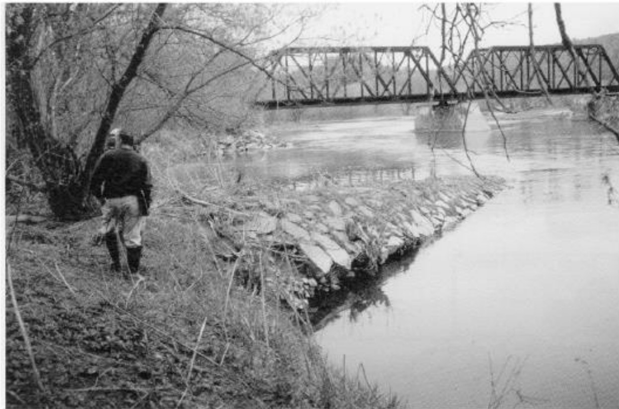
Figure 22. Stream jetty placement for bridge protection
