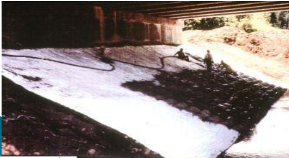
Figure 9.23. Example of the use of cable-tied blocks for scour protection. The photograph (taken as part of an NCHRP project) is courtesy of R. Voigt of The University of Minnesota, Minnesota, U.S.A.
