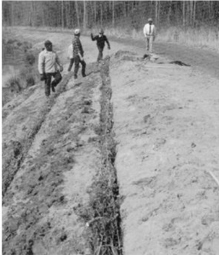
Figure 8. Live fascine placement
