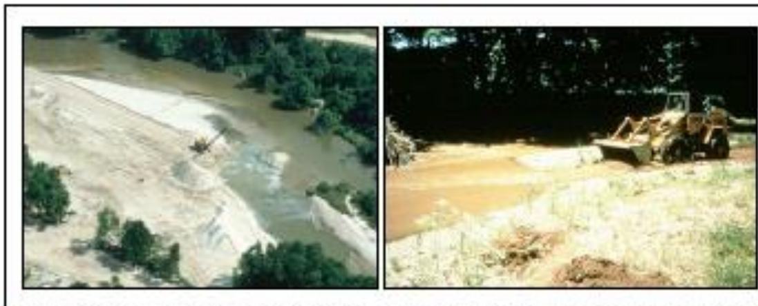
Figure 3.14: Excavating Sand and Gravel from Stream Channels Using Conventional Earth Moving Equipment (Langer, 2003)
