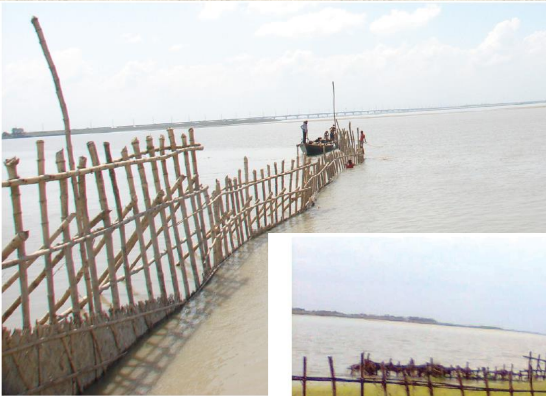
Fig. 3. Bamboo Bandalling in progress in the
