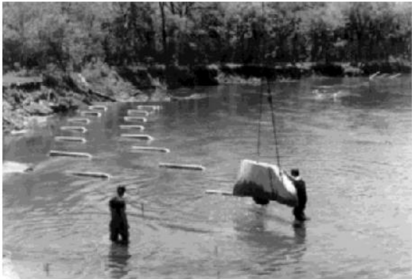
Figure 24. Installation of concrete lowa vanes at low flow
