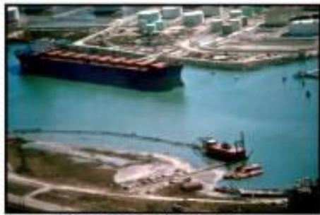
Hydraulic Dredge in Corpus Christi Ship Channel
