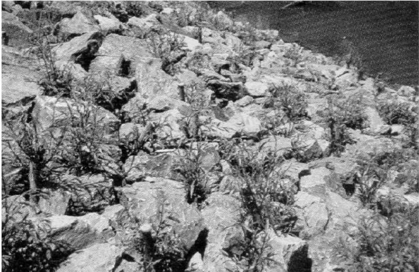
Figure 6. Joint planting system installation
