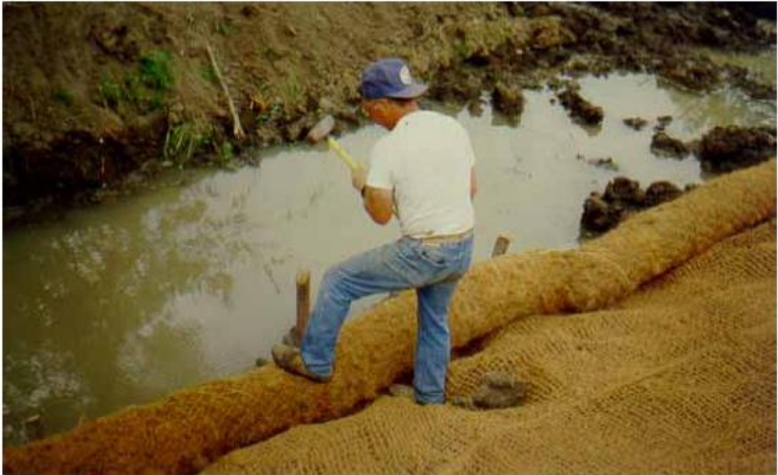
Figure 16. Installation of stakes to secure a coconut roll
