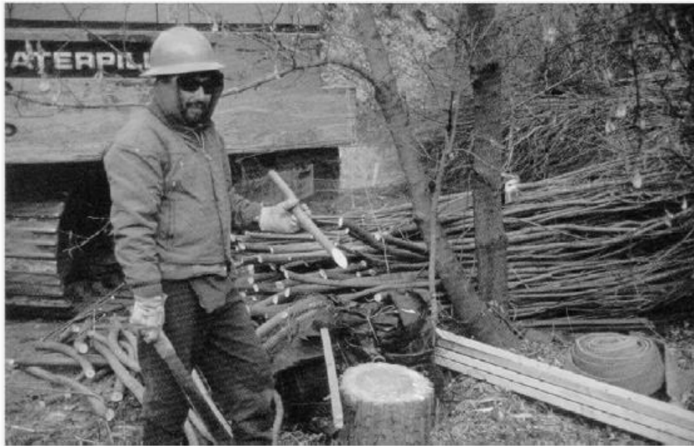
Figure 3. Live stake preparation
