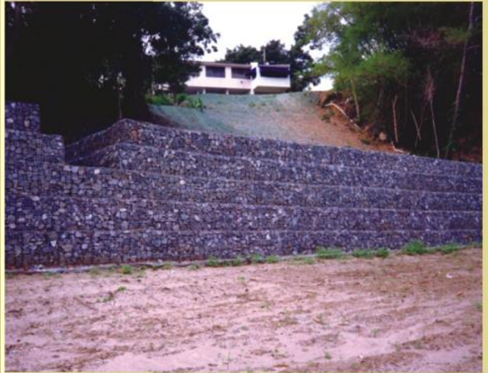
Gabion Gravity Wall
