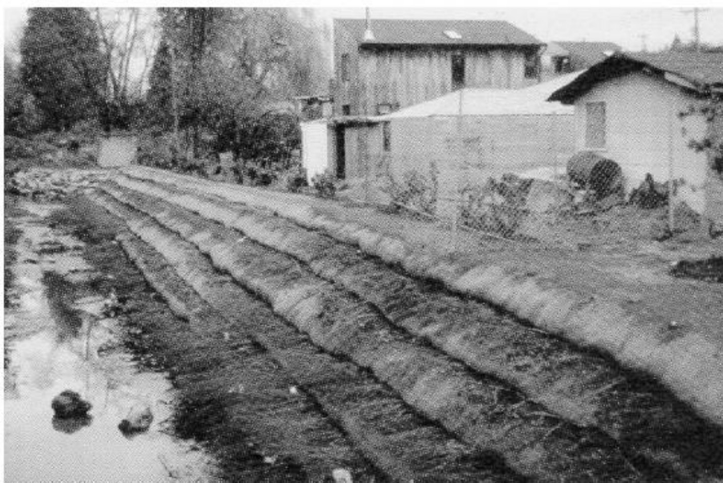
Figure 28. Completed geogrid installation
