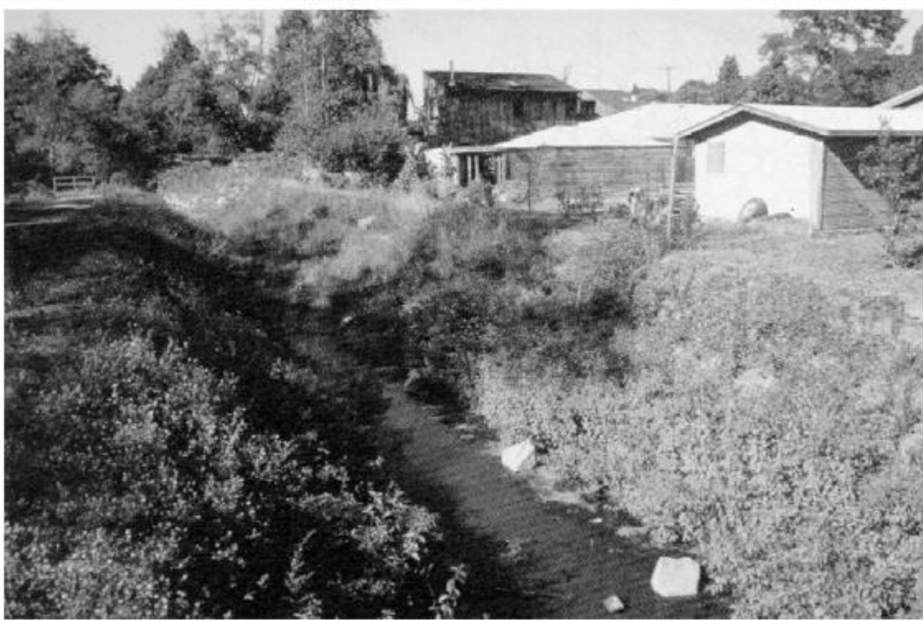
Figure 29. Vegetated geogrid two years after installation
