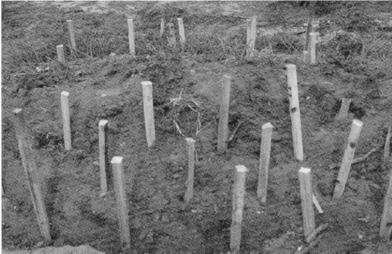
Figure 5. Live stake installation
